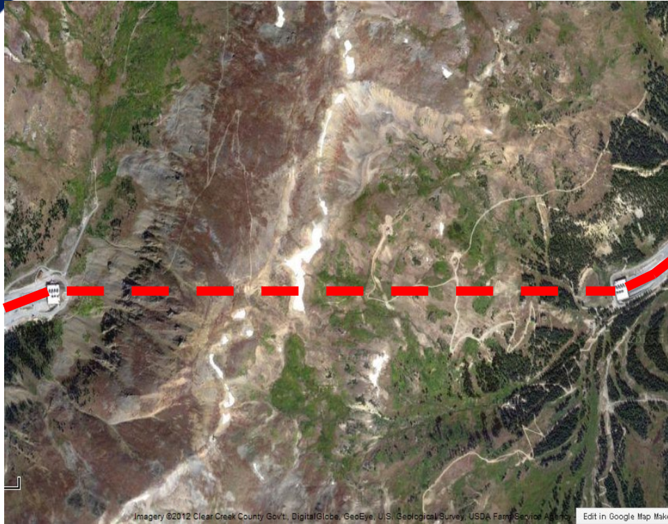
Eisenhower (and Johnson) Tunnels along I-70, west of Denver, CO
